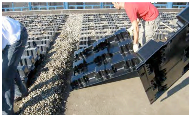
Pose des supports
